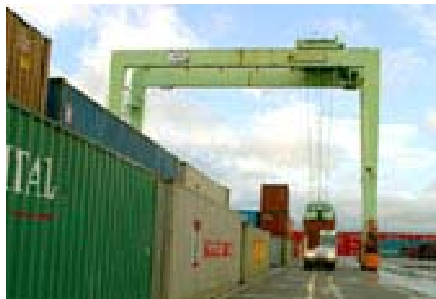
Figure 5.4: Rubber Tired Gantry Crane
