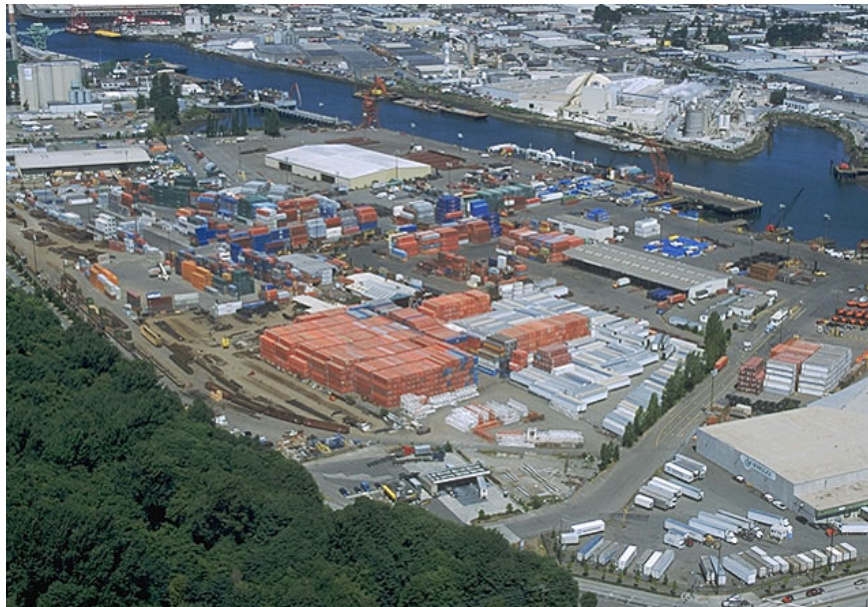
Figure 1.12: Port of Seattle Terminal 115
