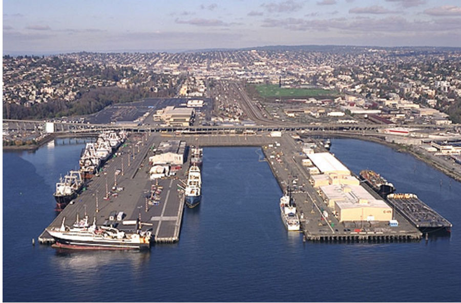
Figure 1.11: Port of Seattle Terminal 90/91
