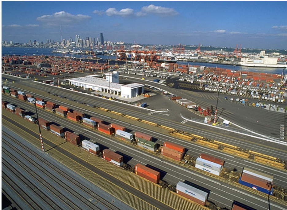
Figure 1.9: Port of Seattle Terminal 5
