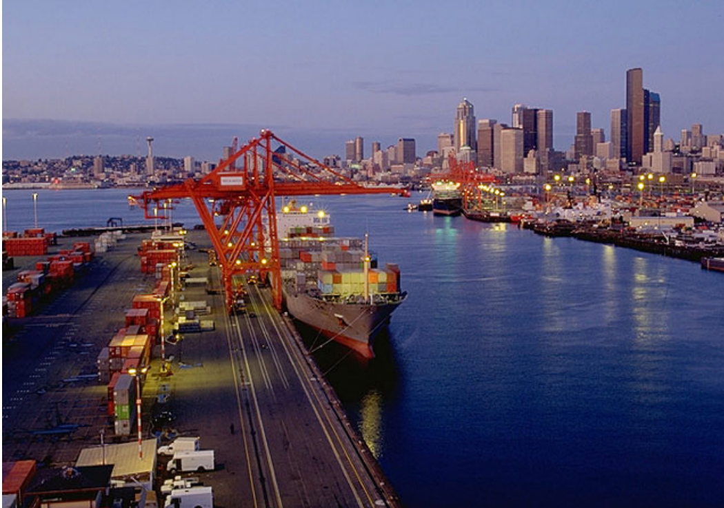
Figure 1.10: Port of Seattle Terminal 18
