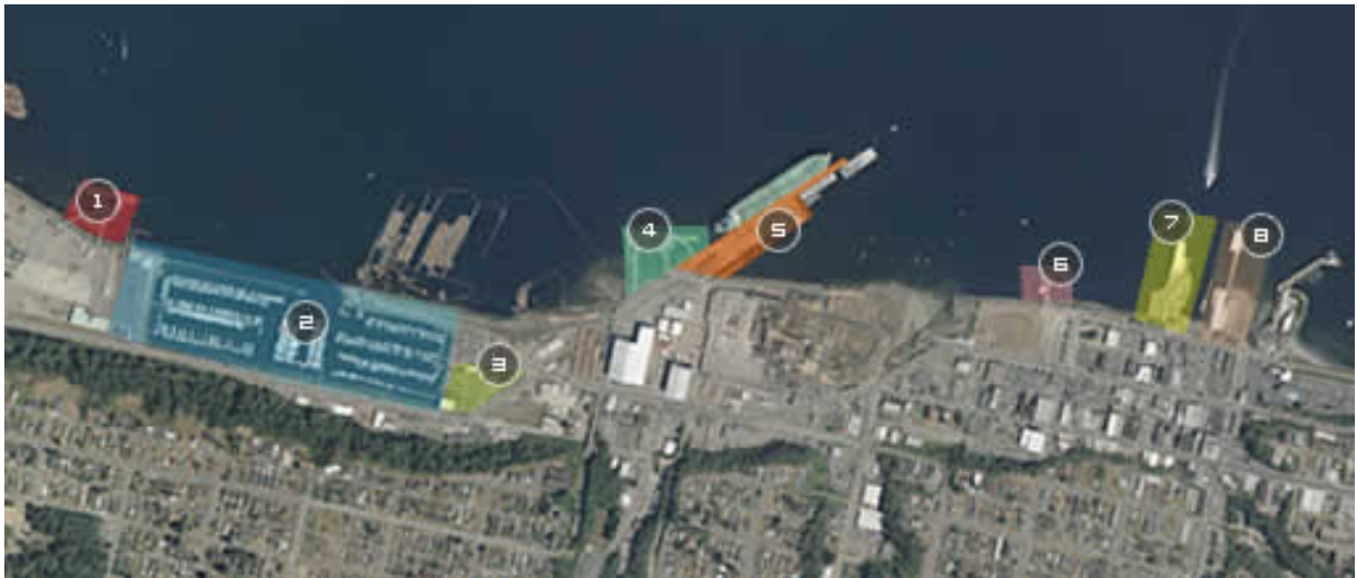
Figure 1.20: Port of Port Angeles Overview
