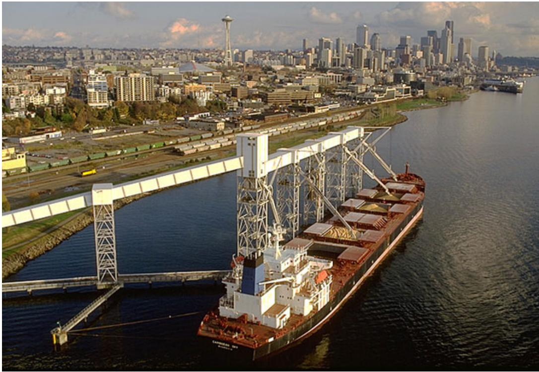
Figure 1.13: Port of Seattle Grain Handling Facility
