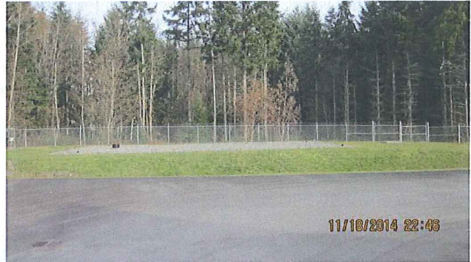
PHOTO #:19 DATE: NOVEMBER 19, 2014 TAKEN BY: CARL JONES DESCRIPTION: BIOFILTER FOR ODOR CONTROL
