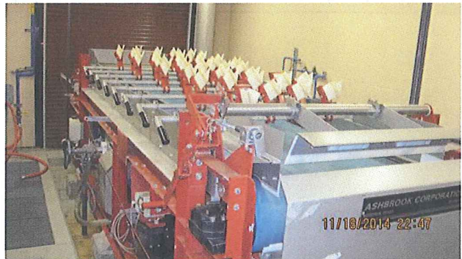
PHOTO #:17 DATE: NOVEMBER 19, 2014 TAKEN BY: CARL JONES DESCRIPTION: GRAVITY BELT THICKENER (GBT)
