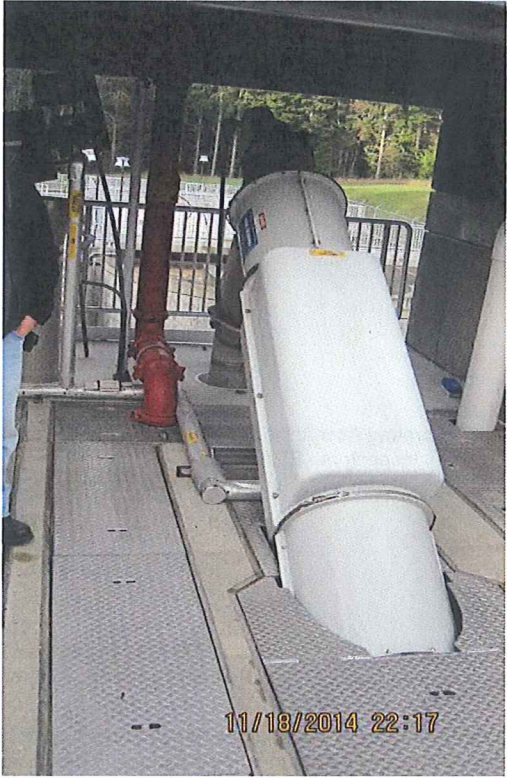
PHOTO #:01 DATE: NOVEMBER 19, 2014 TAKEN BY: CARL JONES DESCRIPTION: HEADWORKS – ROTARY FINE SCREEN
