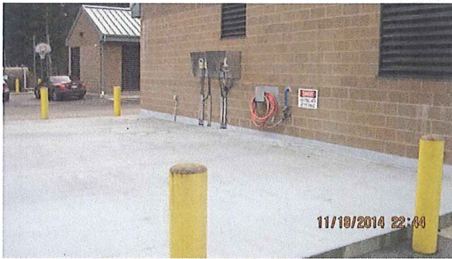
PHOTO #:16 DATE: NOVEMBER 19, 2014 TAKEN BY: CARL JONES DESCRIPTION: WAS AND TWAS STORAGE TANKS (UNDERGROUND)
