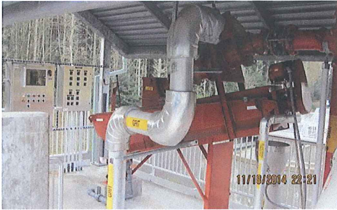
PHOTO #:03 DATE: NOVEMBER 19, 2014 TAKEN BY: CARL JONES DESCRIPTION: HEADWORKS - GRIT CLASSIFIER
