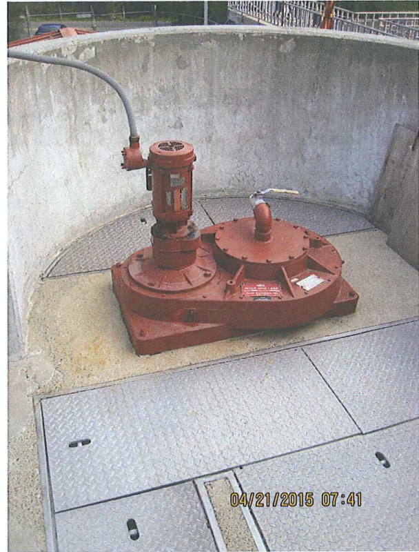
PHOTO # 4 DATE: 04/21/2015 TAKEN BY: LAZARO ELEUTERIO DESCRIPTION: GRIT REMOVAL CHAMBER
