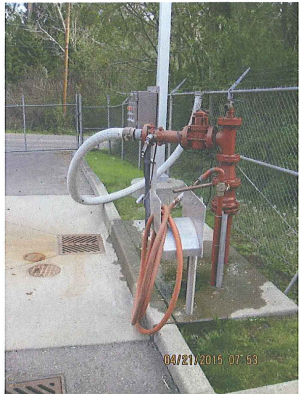
PHOTO # 30 DATE: 04/21/2015 TAKEN BY: LAZARO ELEUTERIO DESCRIPTION: TWAS LOADING TRUCK STATION
