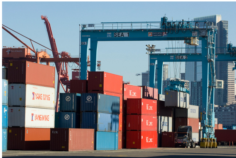
Figure 5.4: Rubber Tired Gantry Crane
